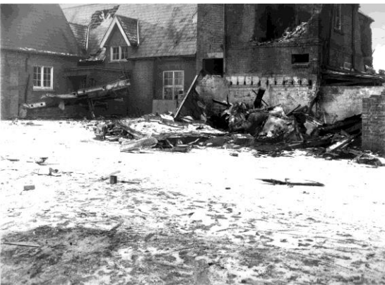
18 th Jan 1946 Wreckage of aircraft and damage to the Headmaster's House at Cove Junior School
